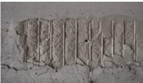
The standard DIN EN 206 assumes concrete structural components to have a service life of at least 50 years. Corrosion of the steel reinforcement in ferroconcrete caused by its exposure to CO<sub>2</sub> (carbonation) can shorten the service life. Holcim HüttenZement GmbH is using a Memmert ICH C climate chamber with CO<sub>2</sub>...
